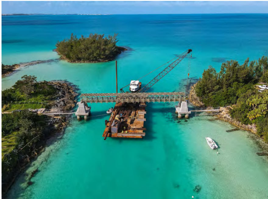
Figure C1.1-1—Flatt's Inlet FRP Pedestrian Truss Bridge (Bermuda) (Source: Creative Composites Group)
