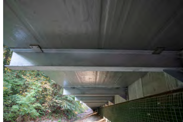
Figure C1.1-5—VIP-Molded FRP Panels Used in Construction of Cantilevered Sidewalk (Arlington, WA) (Source: Francis Zera Photography)
