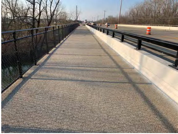
Figure C1.1-4—Pultruded FRP Planks Used in Construction of Cantilevered Sidewalk (Clinton Township, MI) (Source: C.A. Hull Company)
