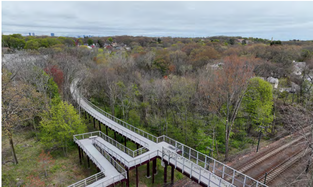
Figure C1.1-3—VIP-Molded FRP Deck Panels Used on Rail Crossing Pedestrian Bridge (Boston, MA) (Source: Creative Composites Group)
