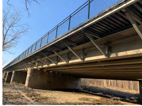
Figure C1.1-4—Pultruded FRP Planks Used in Construction of Cantilevered Sidewalk (Clinton Township, MI) (Source: C.A. Hull Company)
