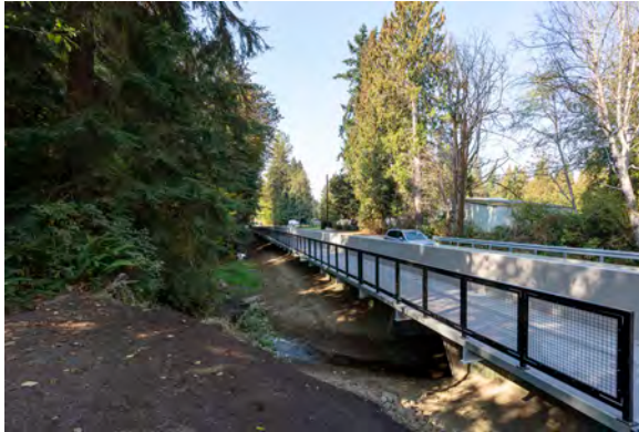
Figure C1.1-5—VIP-Molded FRP Panels Used in Construction of Cantilevered Sidewalk (Arlington, WA) (Source: Francis Zera Photography)
