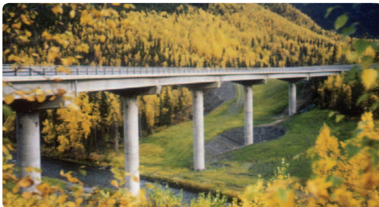
Figure 1-1 Often simply paying attention to proportions and details can result in an attractive bridge with no increase in cost. Canyon Creek Bridge, Anchorage, Alaska.
